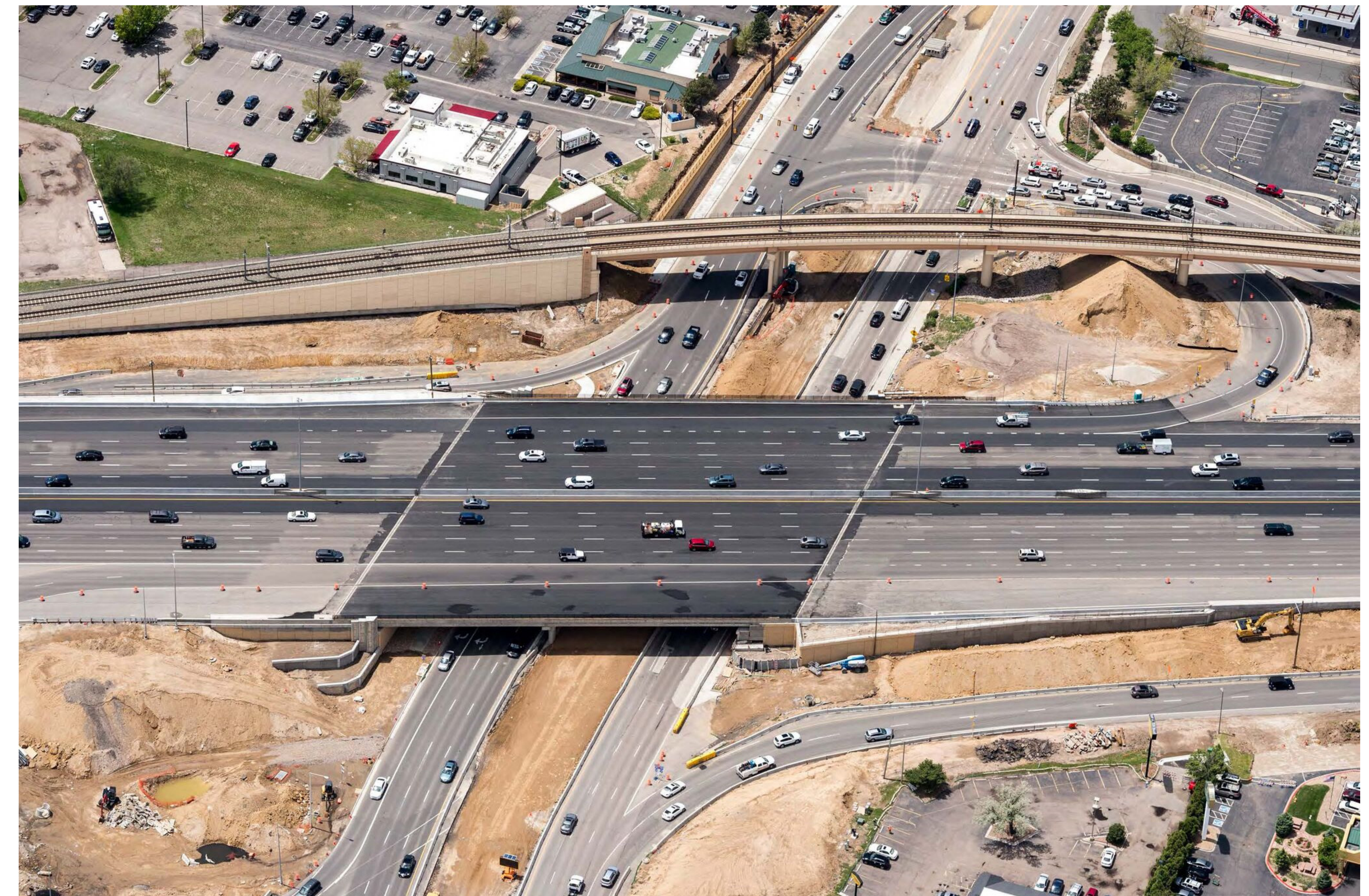
The I-25 and Arapahoe Road Bridge Replacement project used the CM/GC delivery method.
